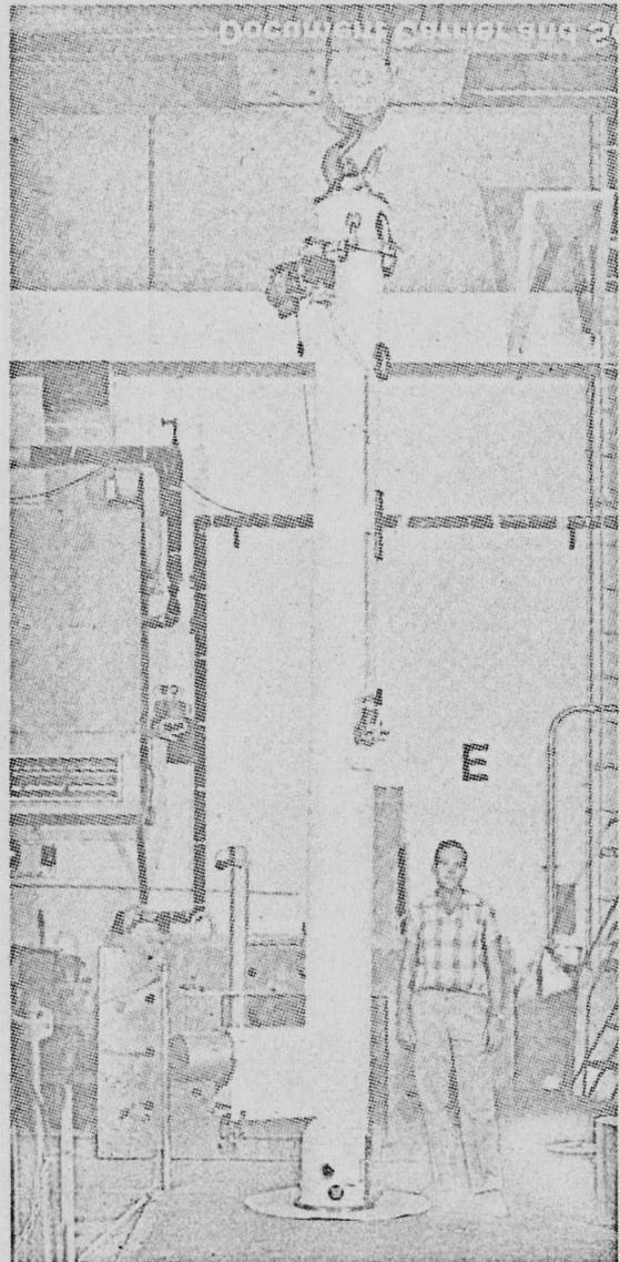
Fig. 3. LAMPRE Fuel Transfer Machine.
