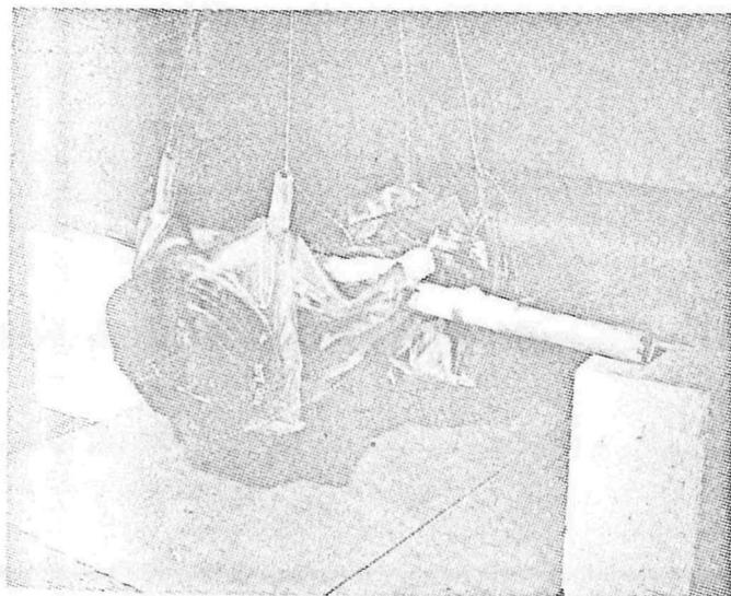
Fig. 12. Typical "Glove Bag" used for Severing Coolant Loop Piping.
