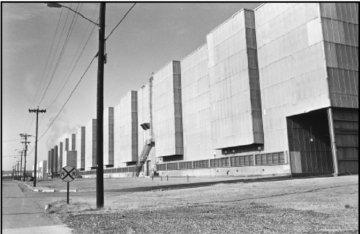
The K-25 Gaseous Diffusion Process Building is half a mile long and 1,000 feet wide. It is comprised of fifty buildings four stories tall and arrayed in a U-shape. The lower floor, which once housed electrical equipment and process control panels, now stores hazardous and radioactive wastes and part of the DOE's stockpile of virgin and enriched lithium. K-25 Process Building, K-25 Gaseous Diffusion Plant, Oak Ridge, Tennessee. January 9, 1994.
