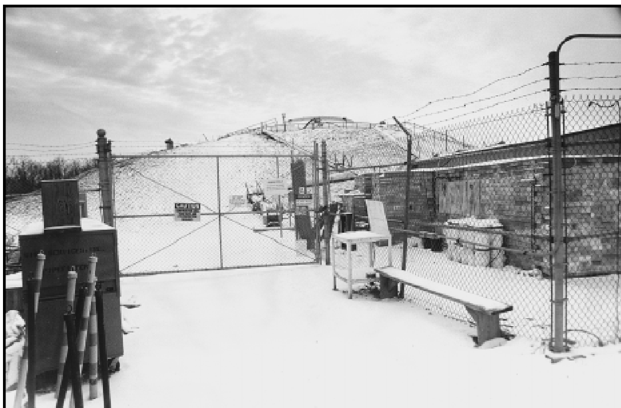
The K-65 Silo. This underground silo at Fernald contains residues from African pitchblende ore refined in upstate New York for the Manhattan Project. The Fernald Plant also placed in this silo wastes from its own uranium processing. Radon gas from this silo and another adjacent to it was the major source of radiation exposure to people in the surrounding area. K-65 Silo, Fernald Environmental Management Project, Ohio. January 29, 1994.
