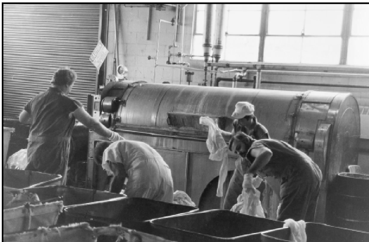
Fernald Laundry. At the Fernald site, over 1,000 pairs of cotton work suits were laundered daily to rid the clothing of uranium dust. Laundry water was treated as low-level radioactive waste because of its uranium content. Feed Materials Production Center, Fernald, Ohio. December 16, 1985.
