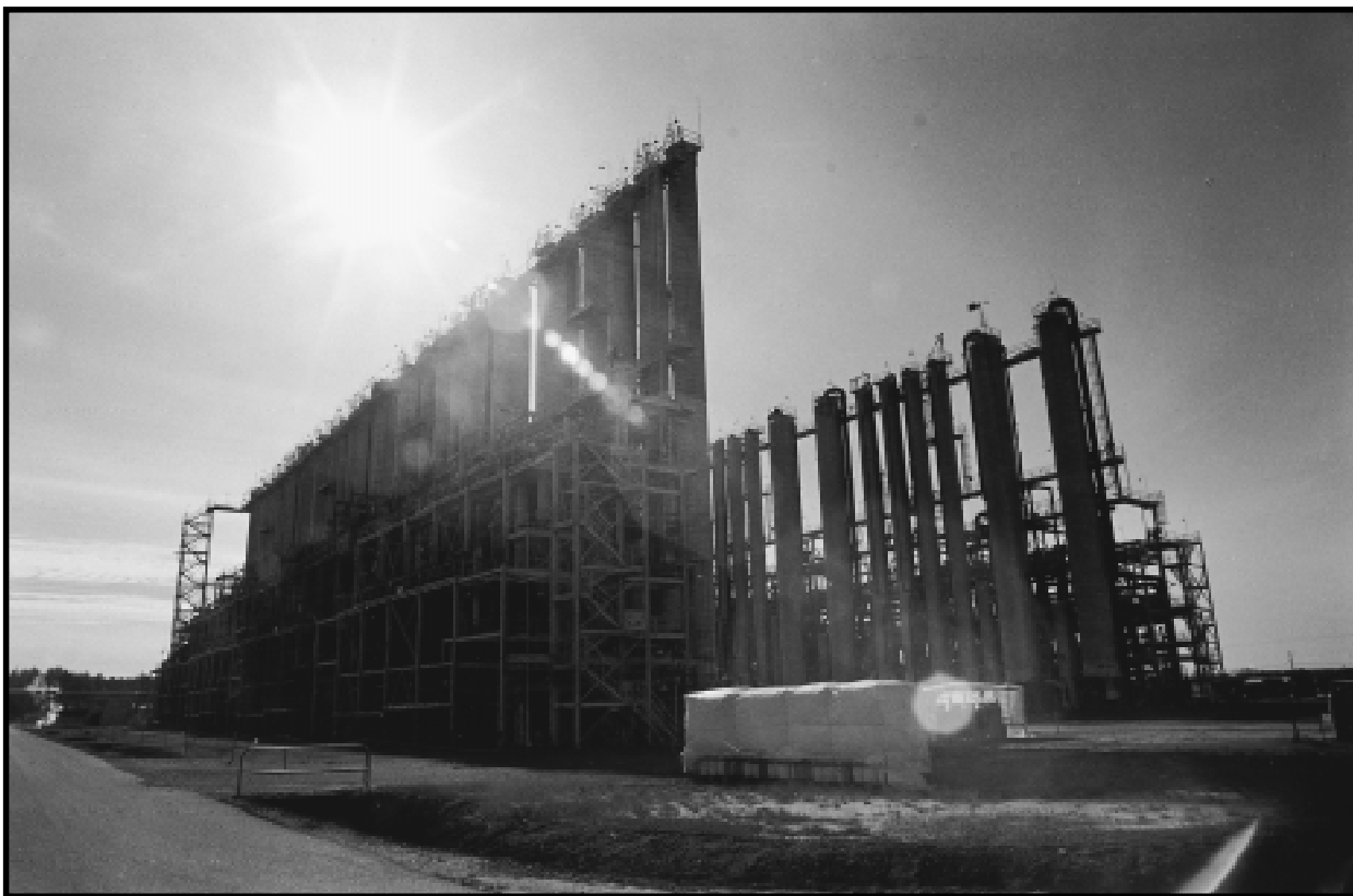
Savannah River Site heavy water facility. For 30 years, this facility concentrated small fractions of heavy hydrogen in natural water to produce some 300,000 gallons of “heavy water” to cool and moderate the site’s five production reactors. Heavy hydrogen extracted at this facility is also used in nuclear weapon components. The facility, built in 1952, has been dismantled. Debris from dismantlement included 180,000 feet of asbestos-covered piping, 150,000 square feet of asbestos-covered equipment, 140 heat exchangers, and 42 towers, each 130 feet tall. Heavy Water Extraction Facility, Savannah River Site, South Carolina. January 8, 1994.
