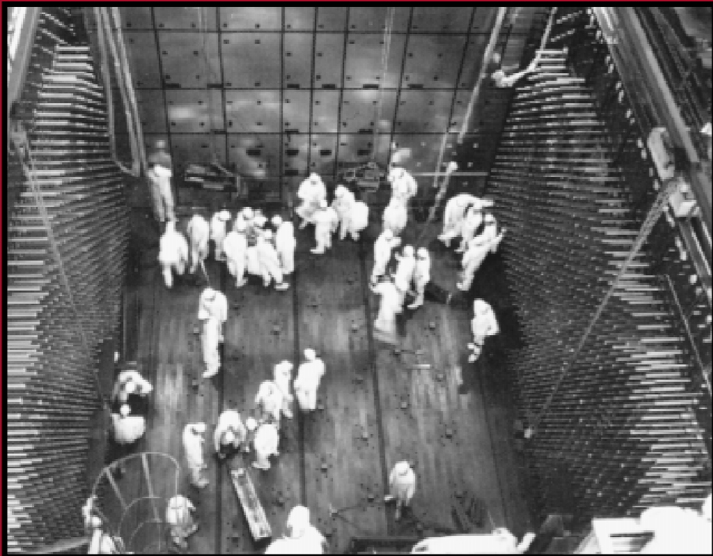
Hanford workers assembling the graphite core of the "C" reactor, 1951.
