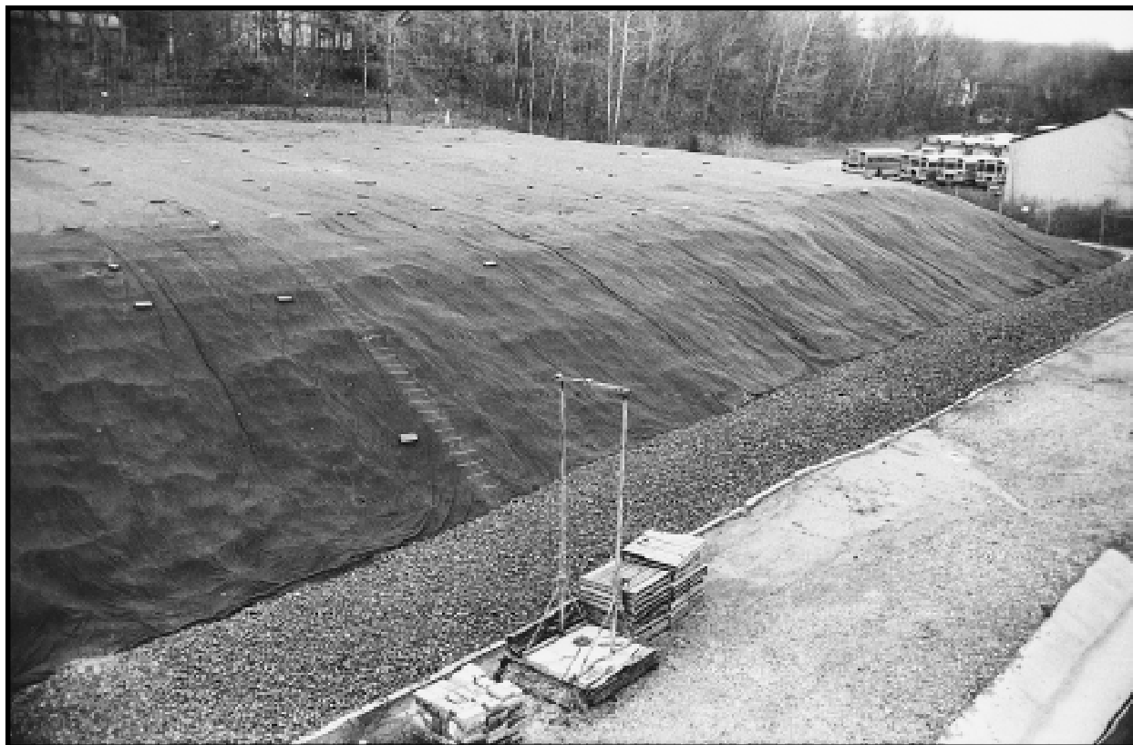
Soil contaminated with uranium residues at the Middlesex Sampling Plant. From 1943 until 1955, most of the uranium purchased by AEC was assayed and sampled at Middlesex. These uranium residues continuously release radon gas. To contain the gas, the soil is covered with an impermeable barrier. Middlesex Sampling Plant, Middlesex, New Jersey. December 10, 1993.
