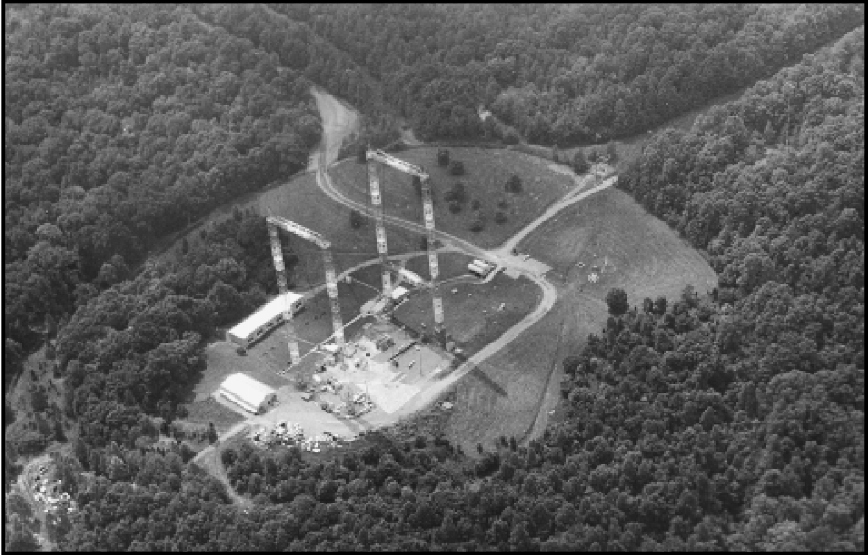
The Tower Shielding Reactor. These towers were built to allow prototype aircraft propulsion reactors to be raised several hundred feet in the air for experiments. A small reactor at the base of the towers provided radiation to measure the shielding properties of materials for weapons and nonweapons programs. Tower Shielding Reactor, Oak Ridge National Laboratory, Tennessee. June 10, 1982.
