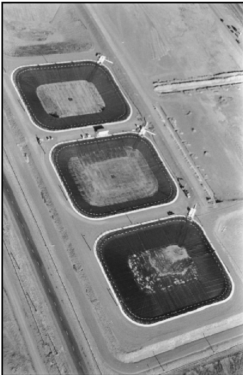
Improving waste management to prevent future contamination. Since 1951, more than 200 million gallons of slightly radioactive water from Hanford's high-level waste tanks were routinely discharged into the soil. Such discharges contributed to Hanford's extensive soil and groundwater contamination. To limit further contamination, Hanford began treating this type of wastewater in April 1994 to remove radionuclides and chemicals before discharging it. Prior to treatment, wastewater is stored in these three 6.5 million gallon, double-lined basins with floating covers and a leachate collection system. Liquid Effluent Storage Facility, 200 Area, Hanford Site, Washington. July 12, 1994.
