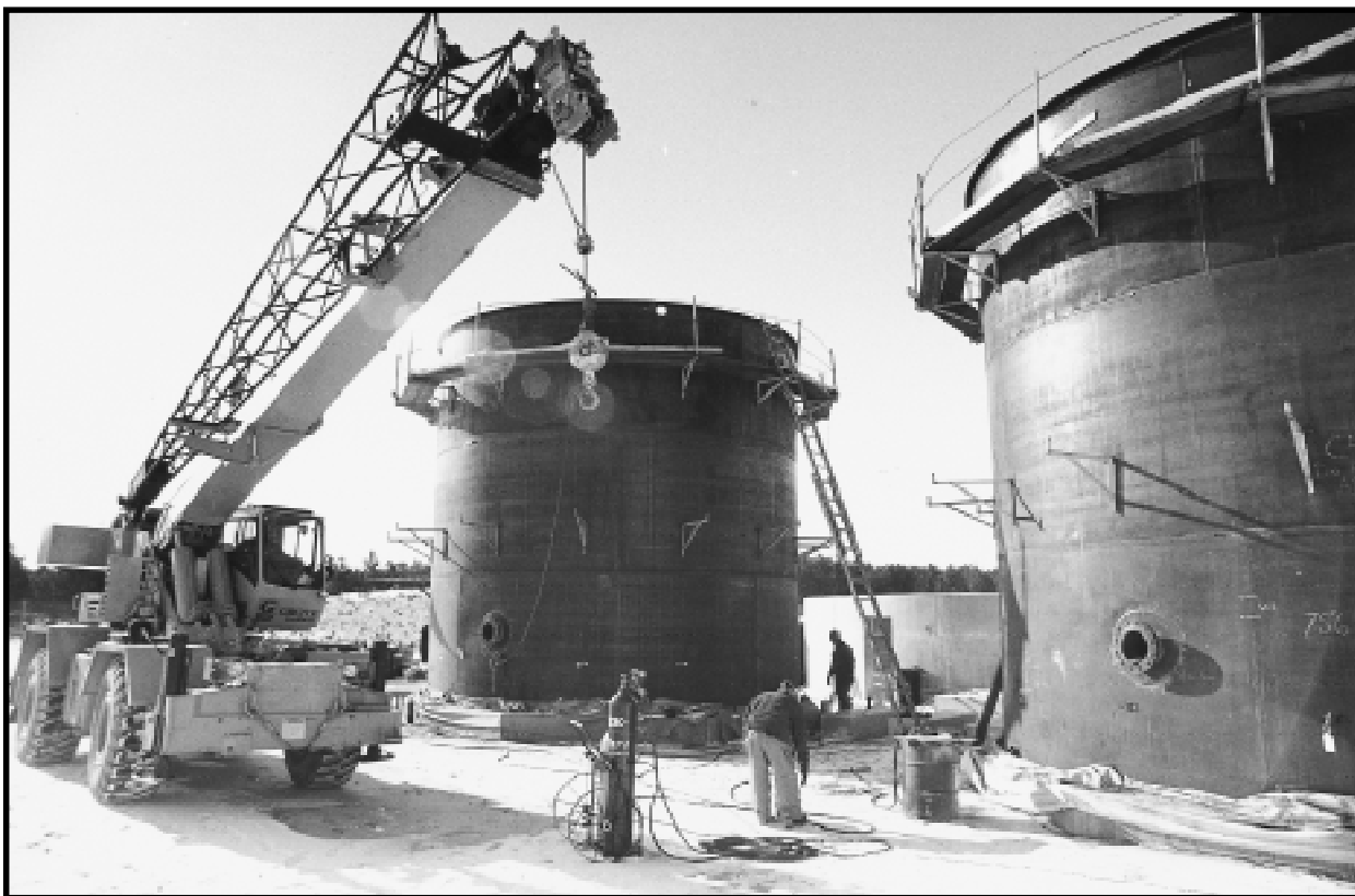
Advanced waste water treatment facility under construction. Fernald Environmental Management Project, Ohio. December 28, 1993.
