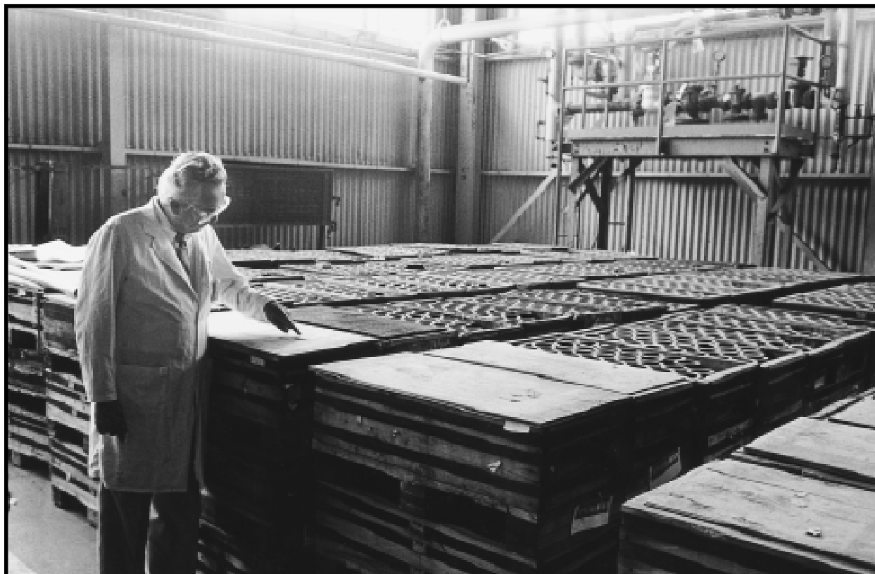
Crates of depleted uranium Mark 31 Target cores await shipment to the Savannah River Site where they would be bombarded with neutrons and partially transformed into plutonium. Fernald Feed Materials Production Center, Fernald, Ohio. December 17, 1985.
