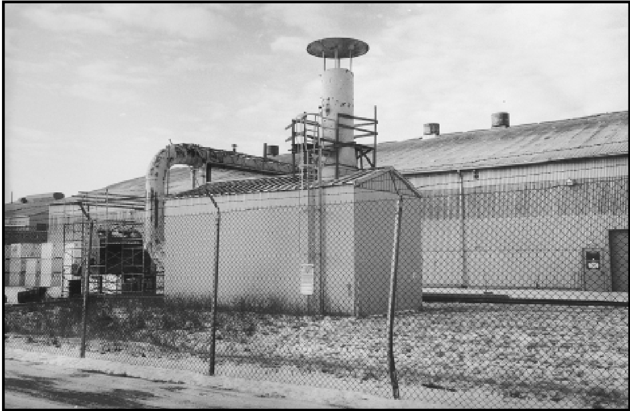
Plant 9 exhaust stack. This exhaust stack was used to control emissions from the Fernald's Plant 9 facility, which processed enriched uranium materials. The malfunctioning of systems like this resulted in releases of several hundred tons of uranium dust to the environment outside the plant buildings over the course of three decades of operations. Fernald Plant, Ohio. December 30, 1993.
