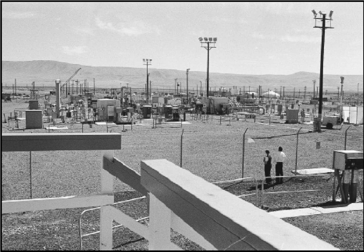
Hanford "Tank Farm." The million-gallon double-walled carbon steel tanks buried here hold high-level nuclear waste from Hanford's plutonium production program. The double-walled tanks have replaced Hanford's older, single-walled tanks which have leaked approximately one million gallons of high-level radioactive waste into Hanford soil. 200 Area, Hanford Site, Washington. July 12, 1994.
