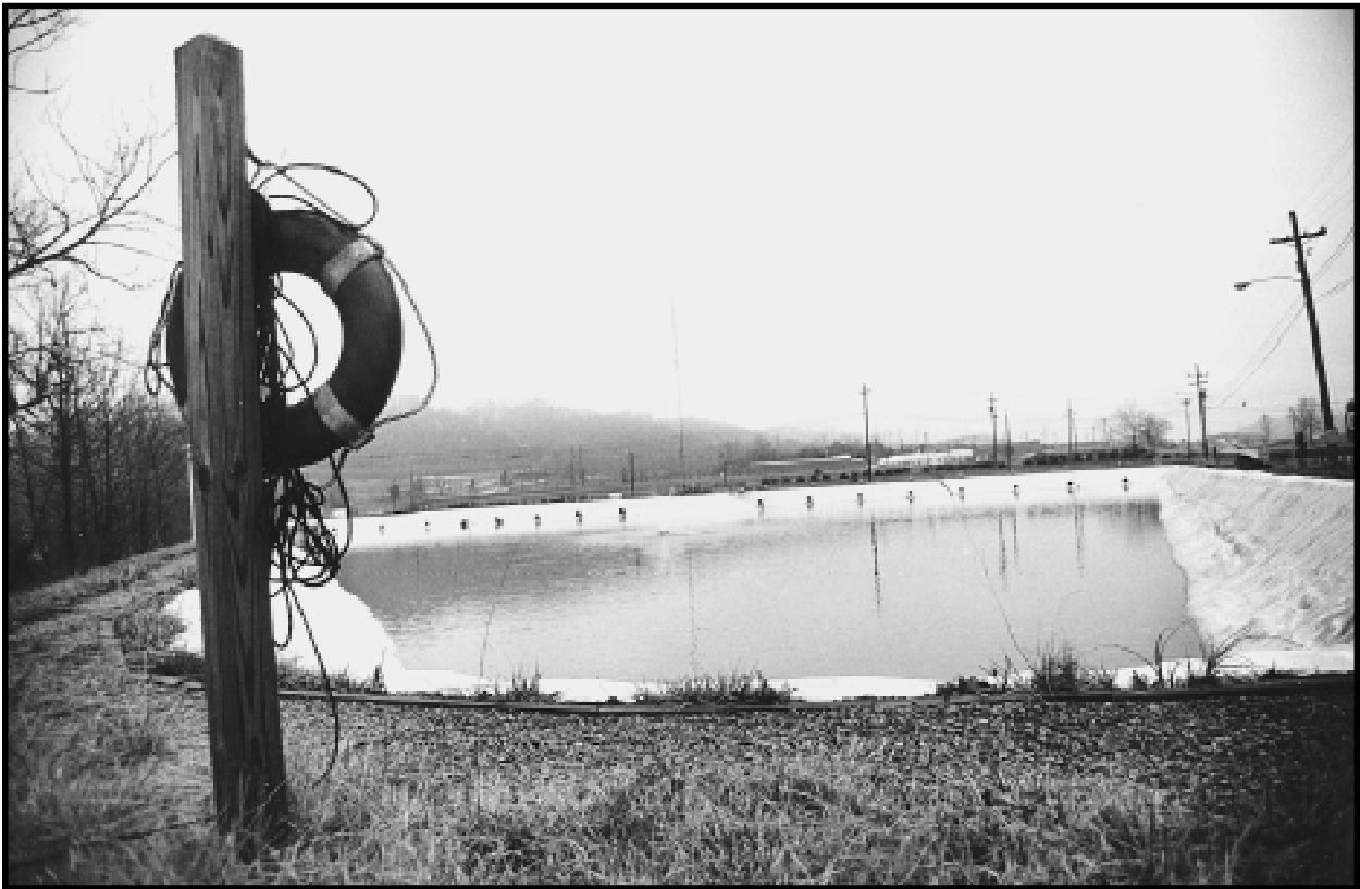
Reality Lake , originally named New Hope Pond, is located at the eastern end of the Y-12 Plant. Engineers created the lake in 1963 to alter the flow of East Fork Poplar Creek, which runs through the Y-12 site. Their aim was to reduce variations in the alkalinity of the creek water and limit the spread of chemical spills. Sediments containing mercury from Y-12 settled at the bottom of the lake rather than washing downstream into the Clinch River. Although this reduced the severity of contamination in the Clinch River system, it poses problems for the environment at Y-12, as the sediments of the creek and lake are severely contaminated. Reality Lake, Y-12 Plant, Oak Ridge, Tennessee. June 15, 1993.
