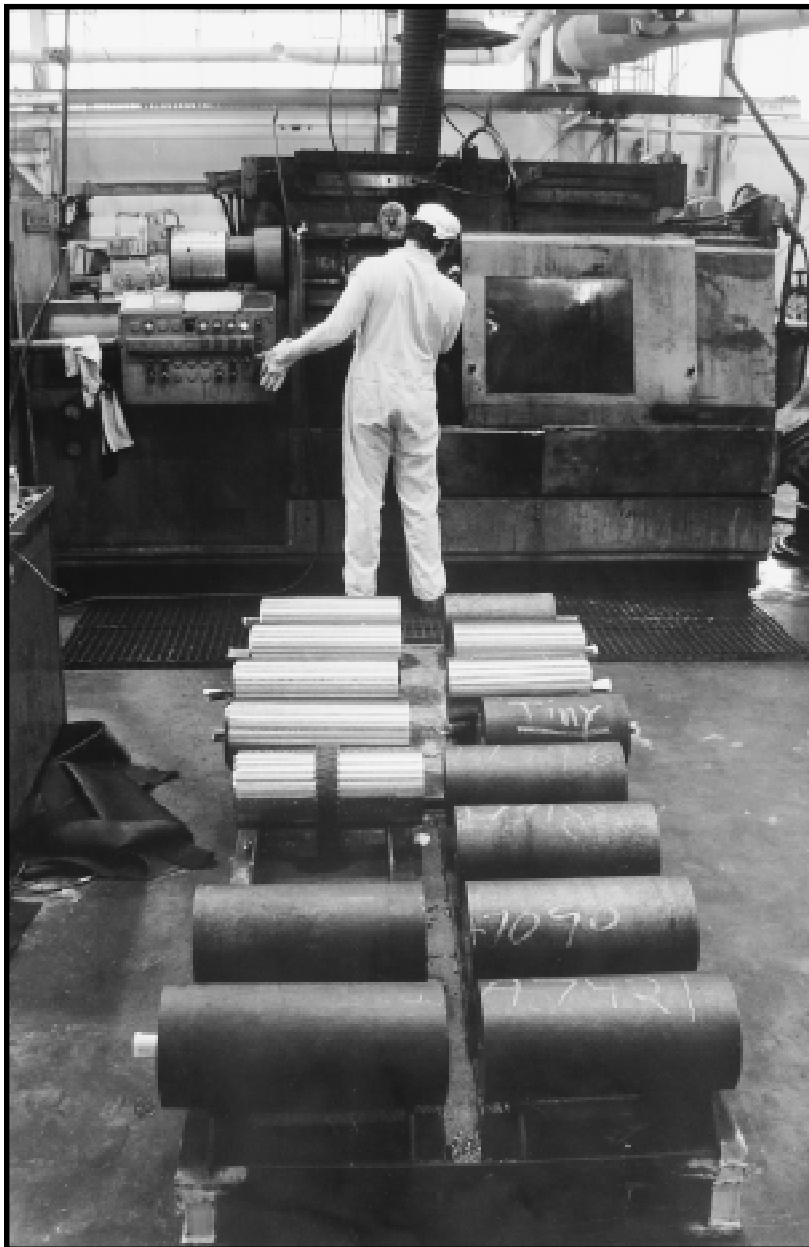
Uranium ingots were machined into billets on a lathe at Fernald. The shiny ingots have been machined while the dull ones have not. Fernald Feed Materials Production Center, Ohio. December 17, 1985.
